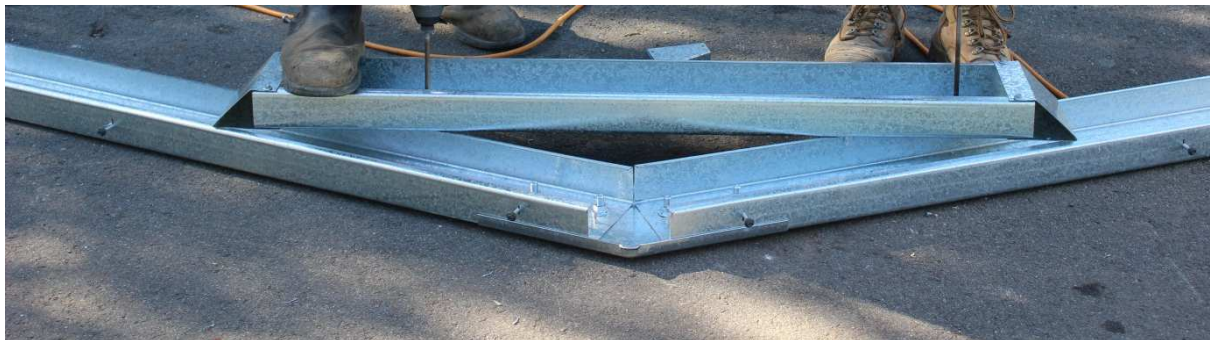
CROSS BEAM ON END BRACKETS TO RAFTER
