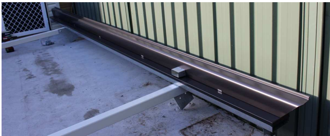
ATTACH BRACKETS TO CLADDING WITH POP RIVETS
