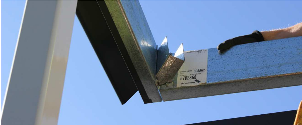
INTERNAL HIP BRACKET TO EAVE PURLIN – BOTTOM VIEW
