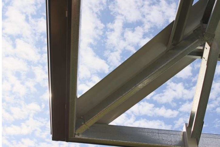
UNDER FLASHING TO DUTCH HIP RAFTER – BOTTOM VIEW
