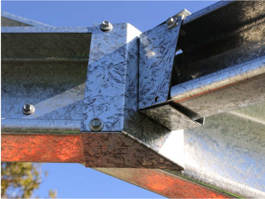
HIP RAFTER TO RAFTER FRAME BRACKET AT HIGH END - CLOSE UP VIEW
